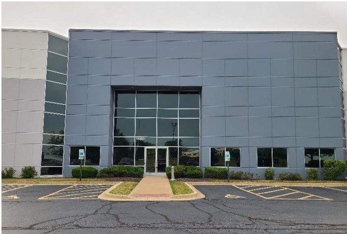
View of North Elevation Toward West
