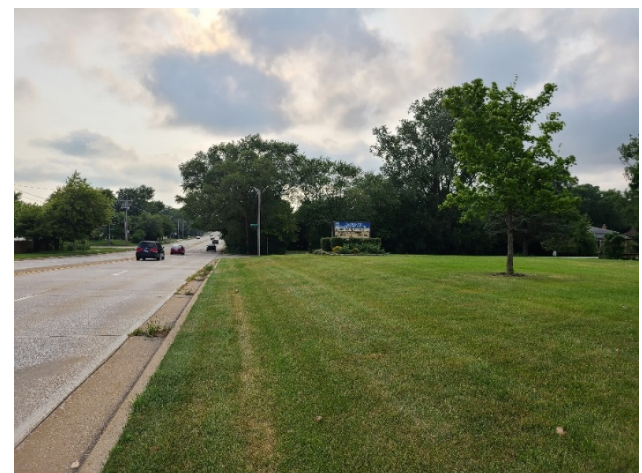
Looking West Showing Sign's Relation to Right-of-Way
